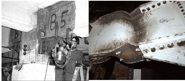
Figure 17: ICF Kaiser bolted connection and test
